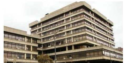
Façade before renovation
