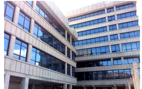
Façade after renovation
